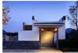
Household Energy Storage
